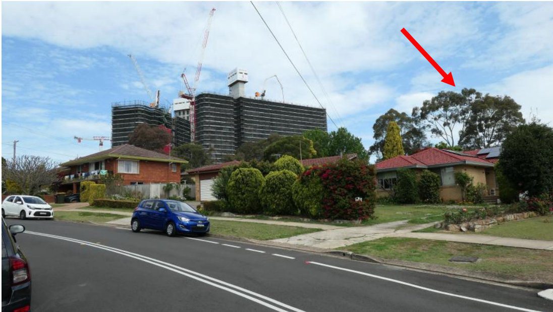
Figure 8 – The site context and trees located on the site that form part of this review. Image taken on Gilham Street looking south towards the high-rise development currently being constructed. The larger trees shown in the right of the image are actually located on the adjoining property to the south. (Source: Arterra– 14 October 2019)
